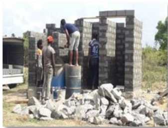
Construction of a house for a vulnerable family- Badulla District
