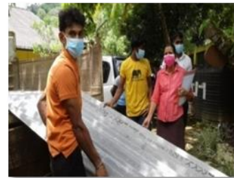
Construction of a tube well – Gampha District
