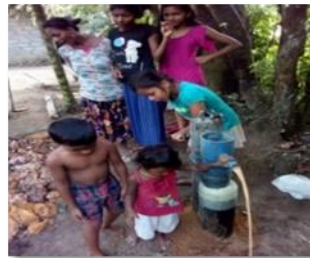
Construction of a tube- well - Gampha District
